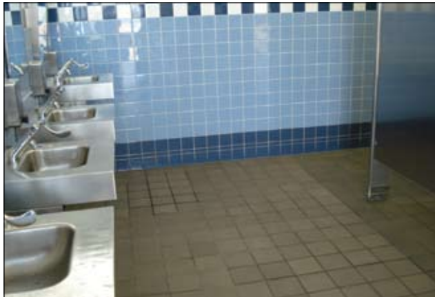
With sufficient resources, all beach bathrooms could be maintained to the standard of this bathroom on South Beach in Staten Island.
