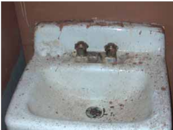
This sink at McKinley Park in Brooklyn is splattered with paint that was never removed.
