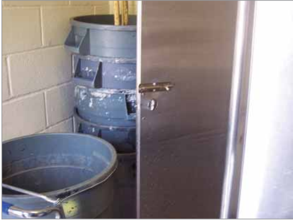
Stored items in this bathroom at Big Bush Park in Queens crowd the area and make it difficult to access the facilities.
